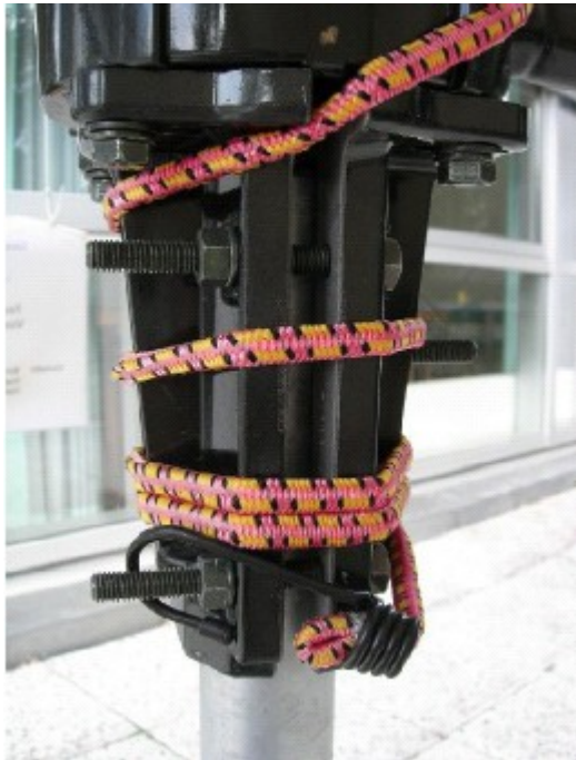
Fig. 10. Rubber Band wrapped around Mast Clamps [Assembly Manual p. 14]
