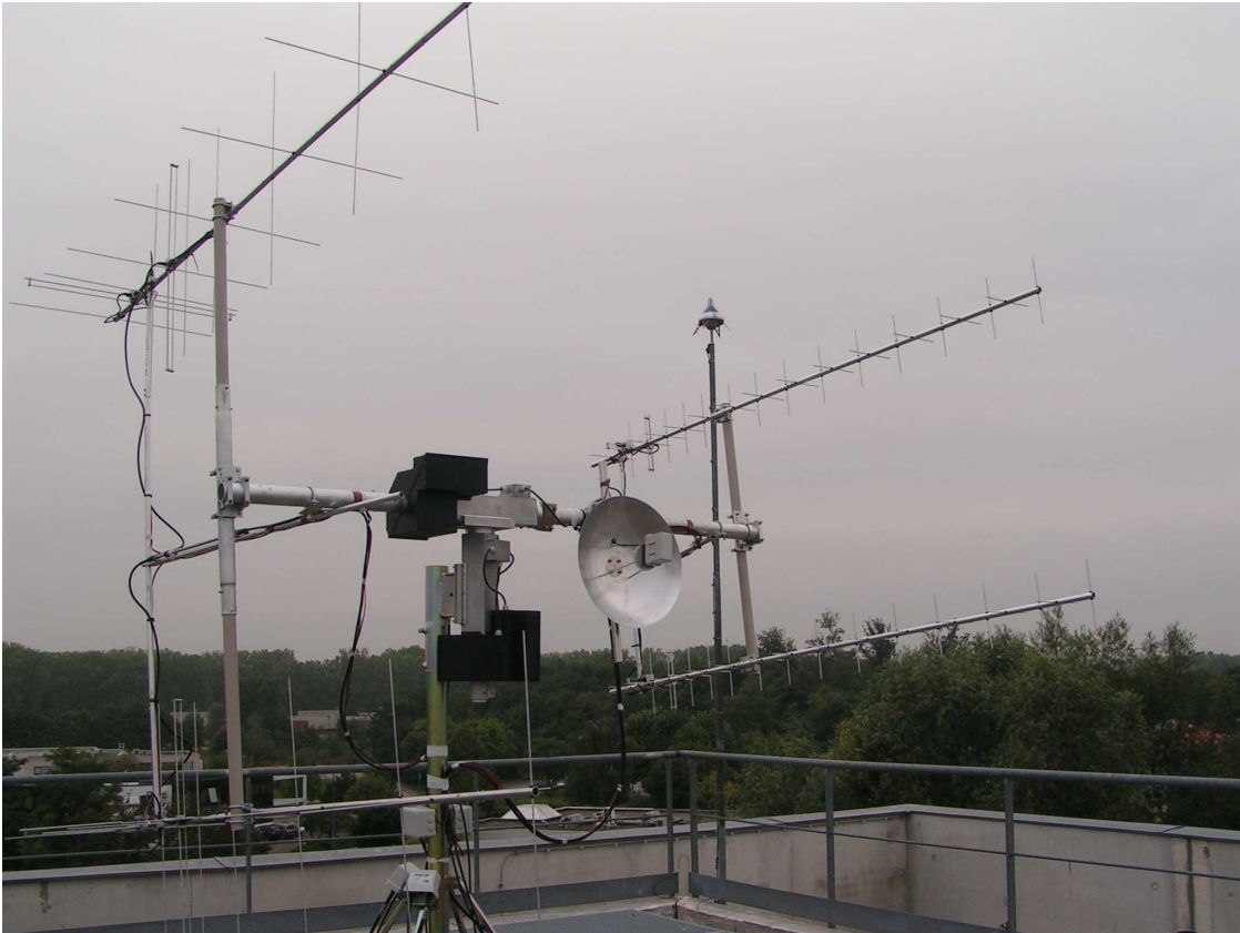
Figure 3.1 The ISU Ground Station antenna system mounted on the ISU building roof.
