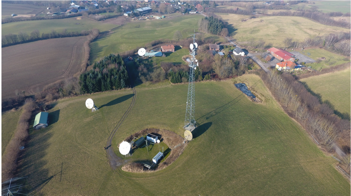
Fig. 2: Overview of the grounds of DLØSHF at the present time: In the background the 9m Sdish for 1.3 GHz, at left the 7.2m dish for 8.4 GHz, at the centre a 7.2m dish for 10 GHz and a 6m dish for 2.4 GHz.
